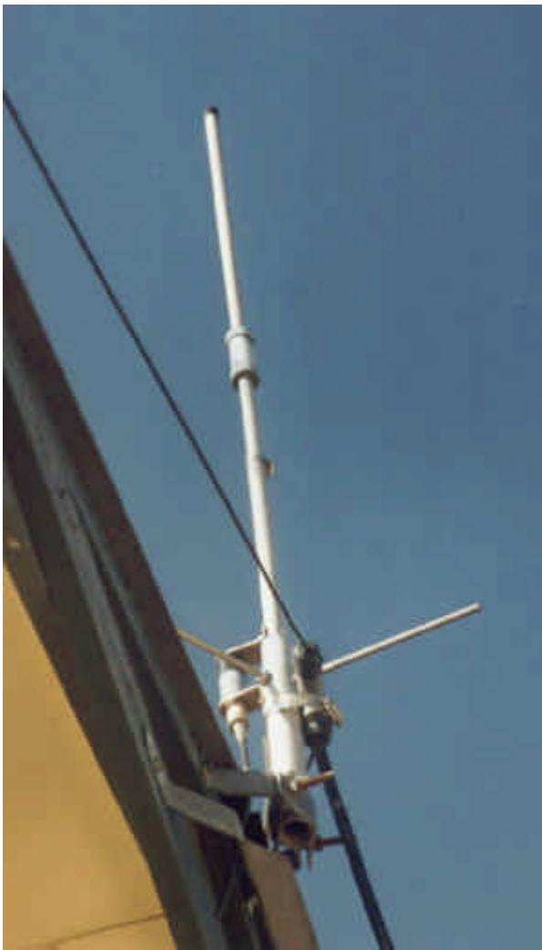
It's not very clear from this photograph, but Steve has a ground wire running from the antenna base down to a 12-ft copper pipe driven into his yard.
