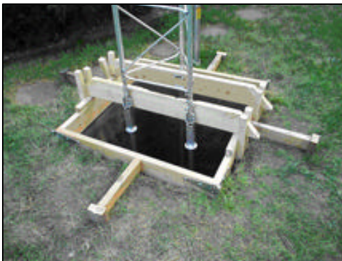
Ready for concrete! (That frame would hold a charging elephant.....make that 7000 pounds of concrete.)
